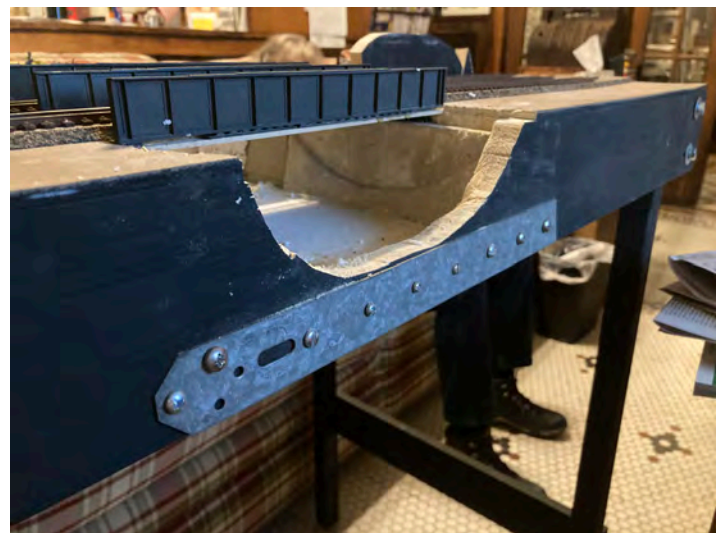
This 3/4 view of the module side shows the steel strap brace that allowed the "digging out" of the module's river.
