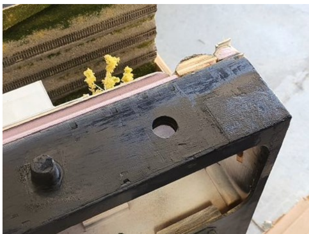
(Pic 11) The completed repair after painting.
